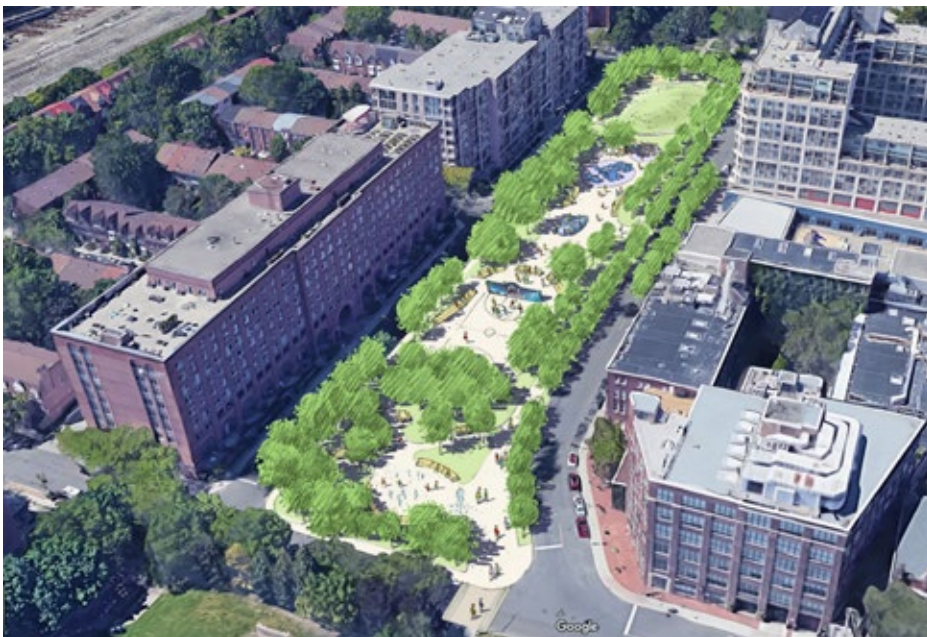
Aerial view of Block 6 showing the water fountain/play area, school yard, and celestial observatory
